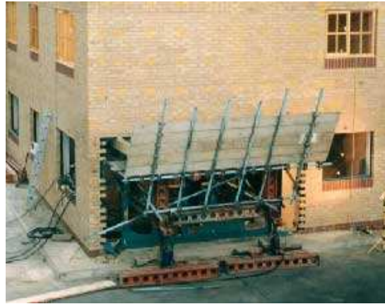
Figure 19. Test of timber frame
