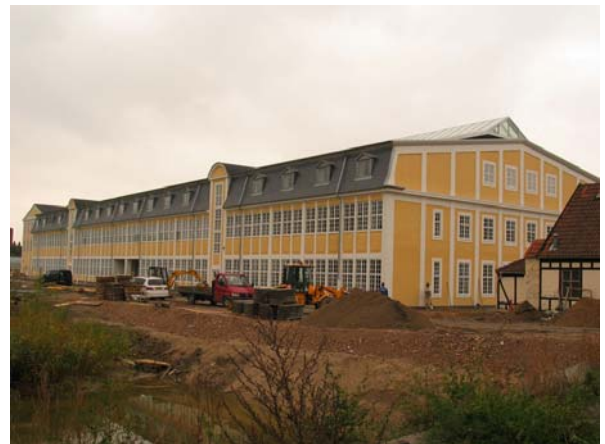
Figure 7. Ovnhallen – being retrofitted.
