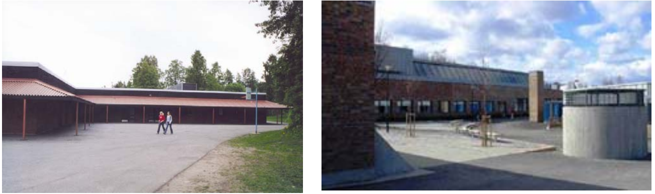
Figure 11. Pictures showing the main building before and after retrofit. The most visible features are the new daylight openings on the roof and new façades. The air inlet tower and a heat recovery unit (roof top) can be seen in the picture to the right. Architects for retrofitting: Hus Arkitekter AS. Photo left: B. Matusiak. Photo right: J. Rolland.
