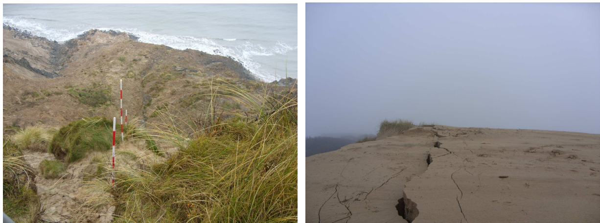
Fig. 1. Left: The slope near Lønstrup after the landslide (December 3rd, 2008). The poles in the photograph are used as points in the land surveying performed. Right: Development of cracks in the sand material (December 3rd, 2008). The photograph is taken approximately 300 metres to the south of the slide.
