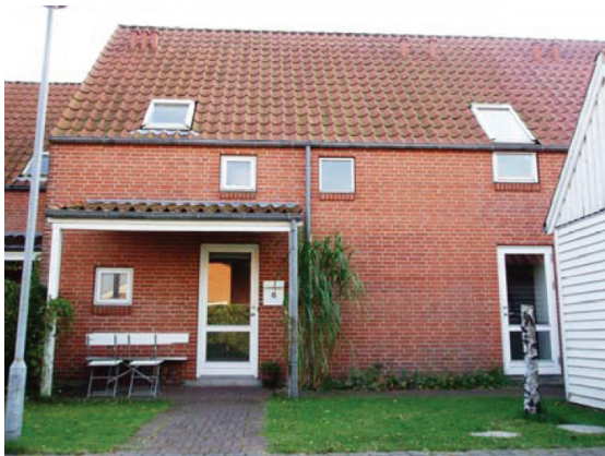
Figure 2 Photo of one of the eight residential buildings.
