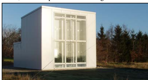
Figure 1. Test facility, 'The Cube'.
