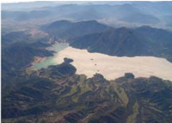
Figure 1: The Caren tailings impoundment at the Codelco-El Teniente Cu mine in Chile.
