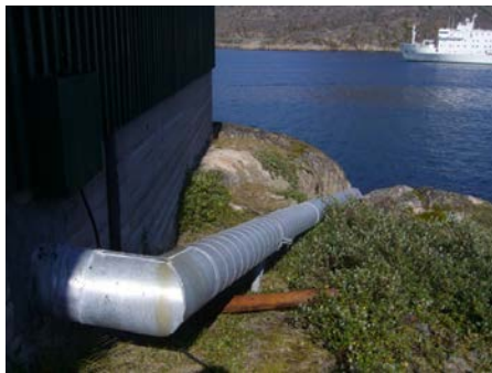
Figure 1: Direct discharge of wastewater to the bay (Sisimiut, Greenland)
