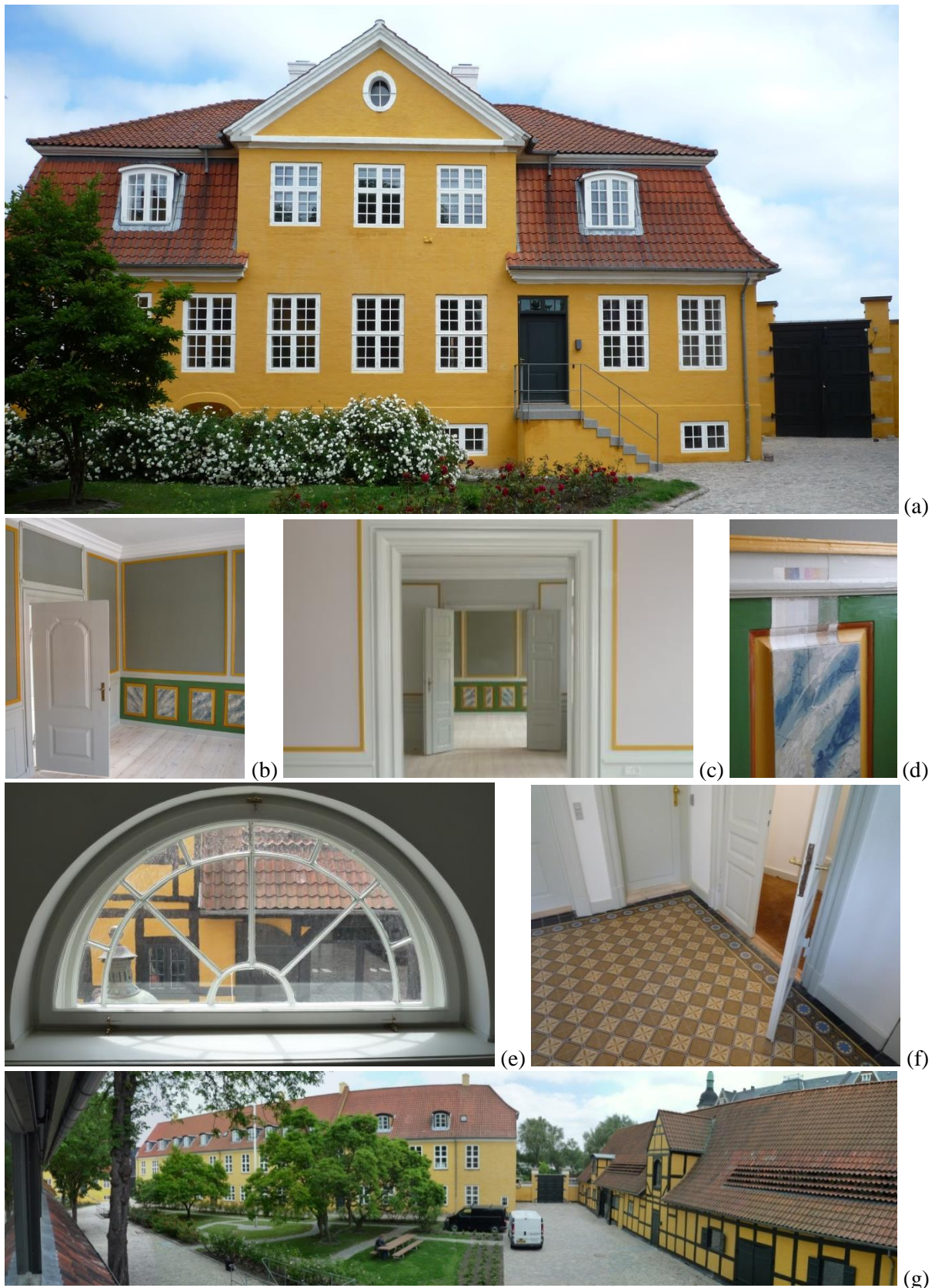
Figure 4. Photos of the refurbished listed complex, Fæstningens Materialgård . a) The supervisor's residence including the photos Figure 4 b) to Figure 4 f), b) Entrance to the main living rooms, c) The living rooms, three rooms in a row lying towards the street, d) Layers of paint found during the restoration and now revealed, e) A window in the staircase, f) The floor-tiles in the entrance hall and staircase, g) Panorama view over the courtyard of the refurbished listed complex, Fæstningens Materialgård .
