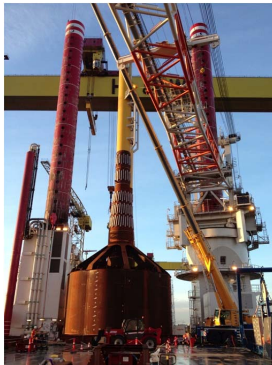
Figure 1: Large-scale monopod bucket foundation on the deck of a jackup vessel
