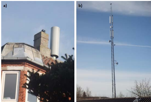
Fig. 1. Typical urban BS deployments considered in the paper: a) rooftop, b) telecommunications tower.
