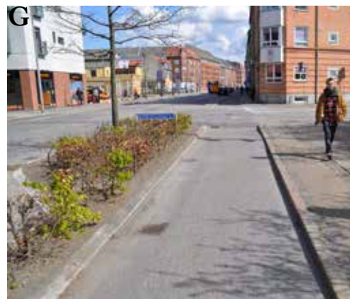
Picture G: When it rains this part of the bicycle lane is filled with water hours after. It is both fun and a little annoying to bike through. There is a risk to get wet feed if you do not lift them.
