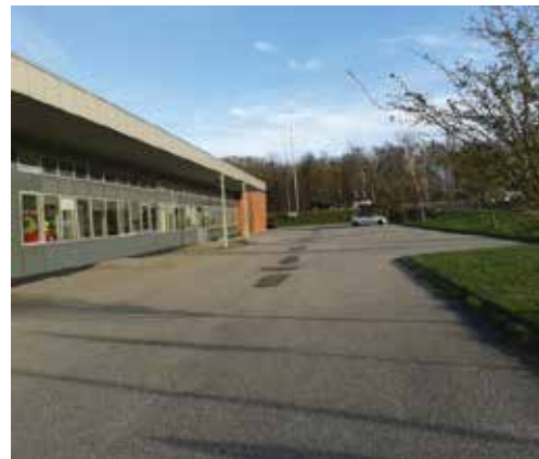
Picture F : When the respondent arrives or departs from work, it is usually dark and the parking lot outside is poorly illuminated. Furthermore there is not much to appeal to the senses, except the view to a forest in the background.
