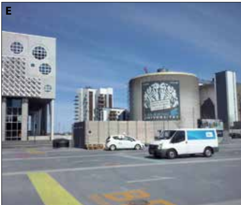
Picture E: The place of encounter between new modern architecture and old water tank creates a heterogeneity in Aalborg. This industrial character still remains in some buildings all over the city, but the contrast with the Musikken Hus captured Gosia's attention. She is not very sure if she likes it, but it is capturing her mind.
