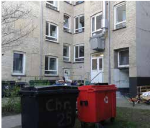
Picture A : This is the back entrance of the respondents house, placed in the courtyard where she can keep her bike. From here she can choose an opening that points in direction of her destination. She experiences the courtyard space as safe, quiet and comfortable, with plenty of daylight, and centrally located in the city. It brings her a sense of relief, as it is a place where she wants to stay and can withdraw from the hassle of her everyday duties.
