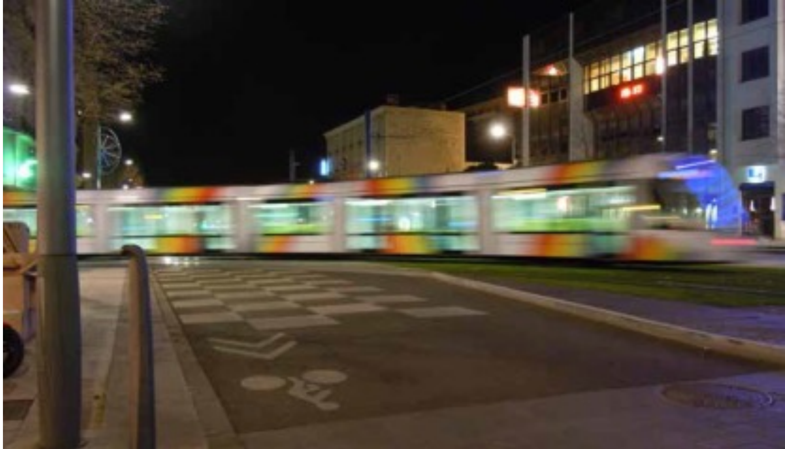
Figure 1 Light rail in Angers, France
