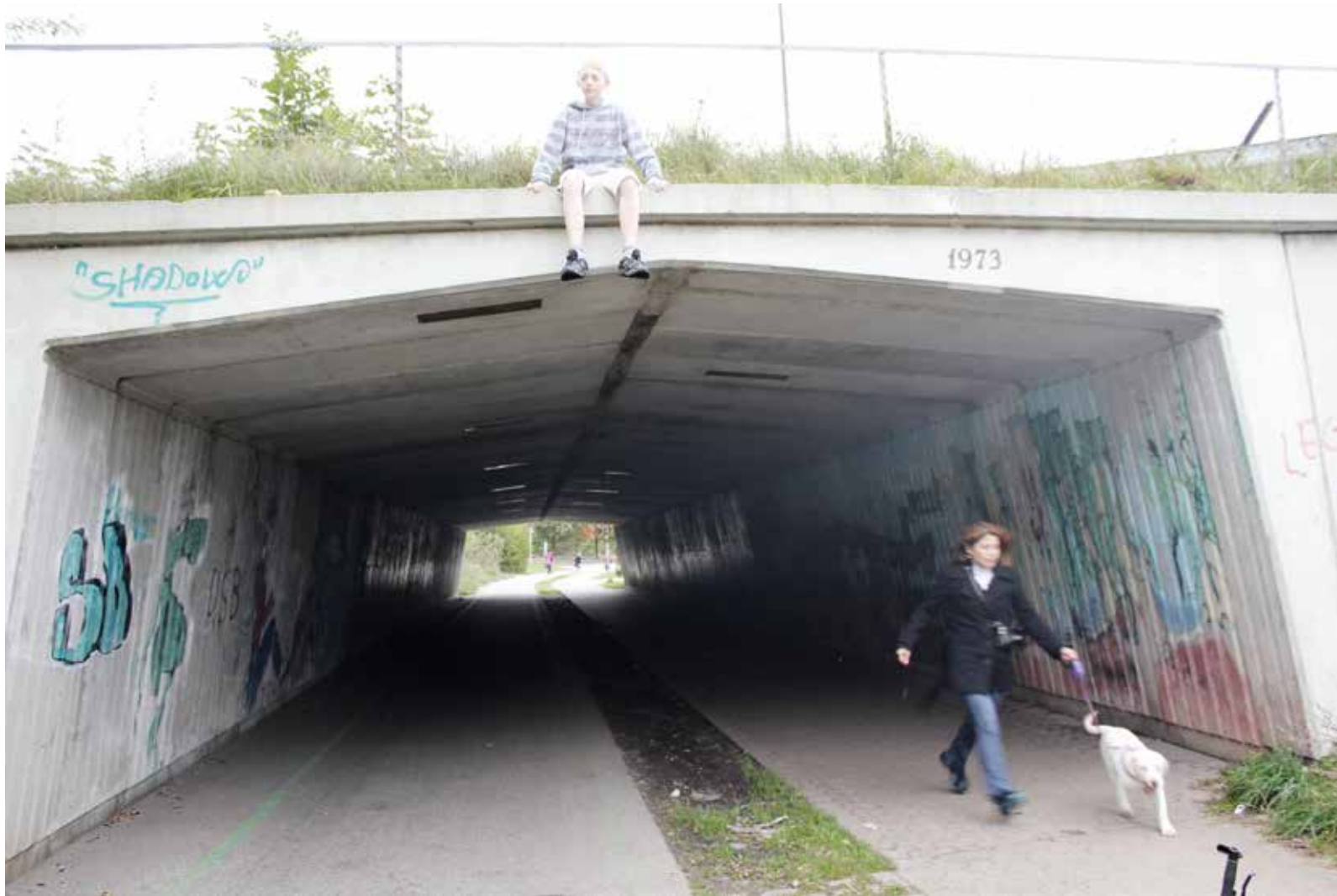
Figure 1: Photo of the tunnel at the study site, Aalborg East
