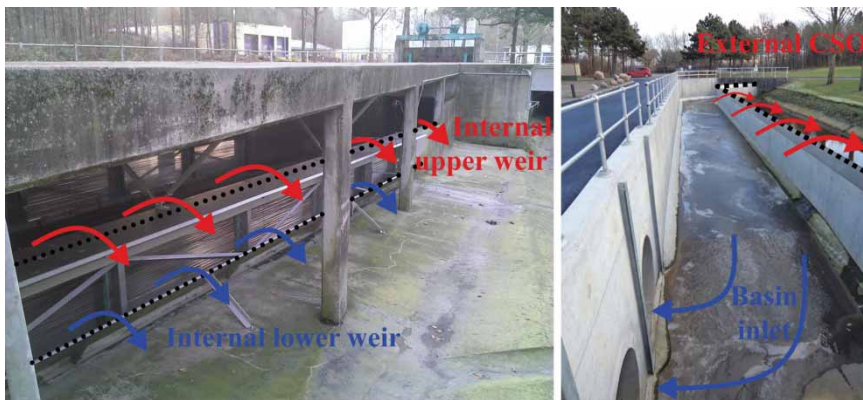
Figure 4 | Photograph of the internal and external CSO during dry weather. The left photograph is taken from the north-eastern side of the internal CSO structure. The internal CSO is symmetric along the centreline of the inflow channel. The right photograph is taken from the western side of the external CSO structure.
