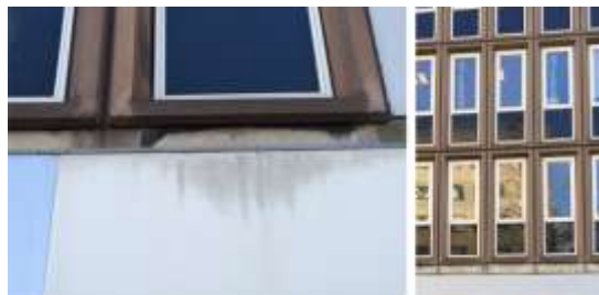
Figure 5: Problems like mould in the façade.
