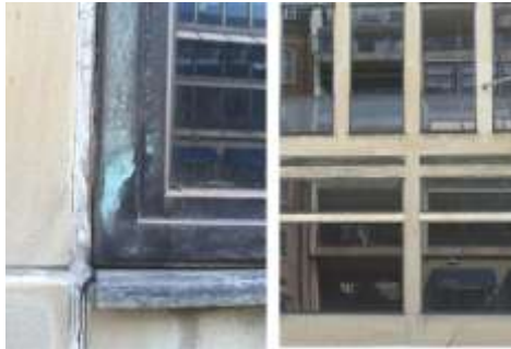
Figure 6: Problems in sealing materials in some parts of the facades.
