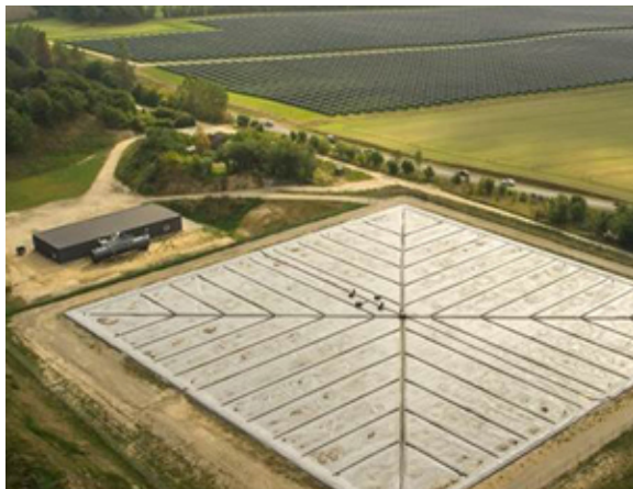
Figure 5.4 PTES connected to solar thermal plant in Dronninglund, Denmark (PlanEnergi 2016)
