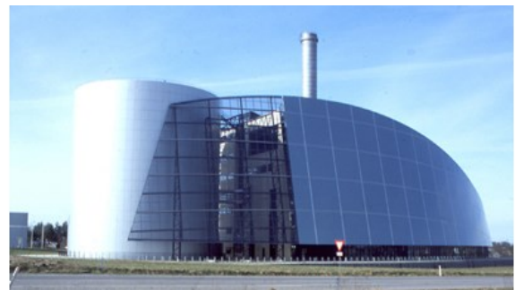
Figure 5.2 CHP plant with connected TTES in Viborg, Denmark (Mørch 2014)
