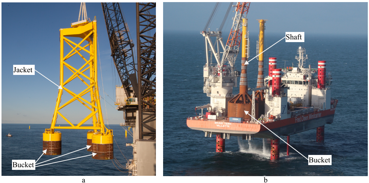
Fig. 1. Offshore wind foundations. (a) Suction bucket jacket. Photo: Courtesy of DONG Energy. (b) Two mono buckets on a jack up vessel for installation. Photo: Courtesy of Universal Foundation Norway.
