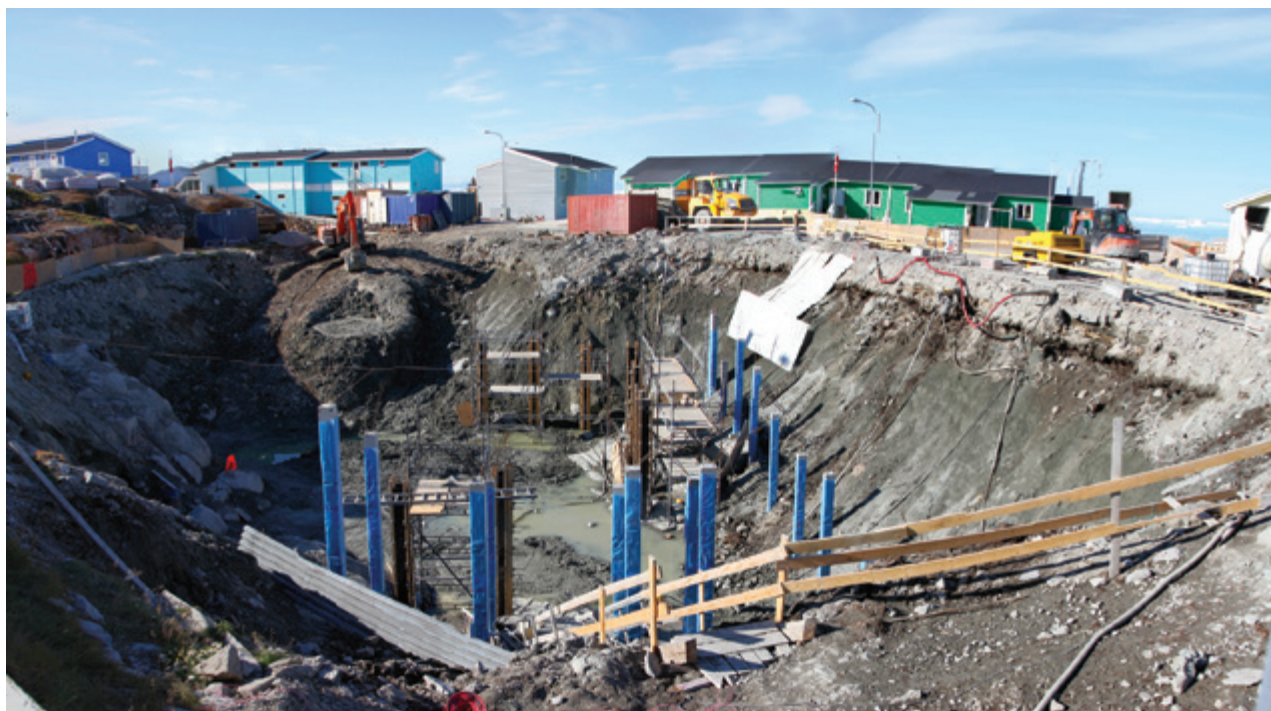
Figure 10.27 Excavation and in situ casting of piles for the new district court house in Ilulissat, August 2015. The photo illustrates the current practice of excavating to bedrock for in situ casting of piles anchored in the bedrock, followed by backfilling (photo by Thomas Ingeman-Nielsen).
