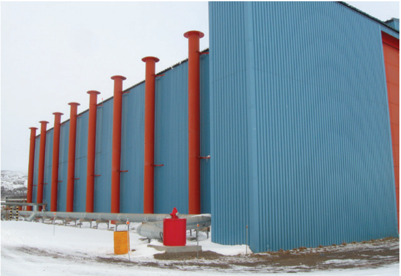
Figure 10.18 Aircraft hangar under-floor cooling plenums, Thule Air Base (photo by Kevin Bjella).
