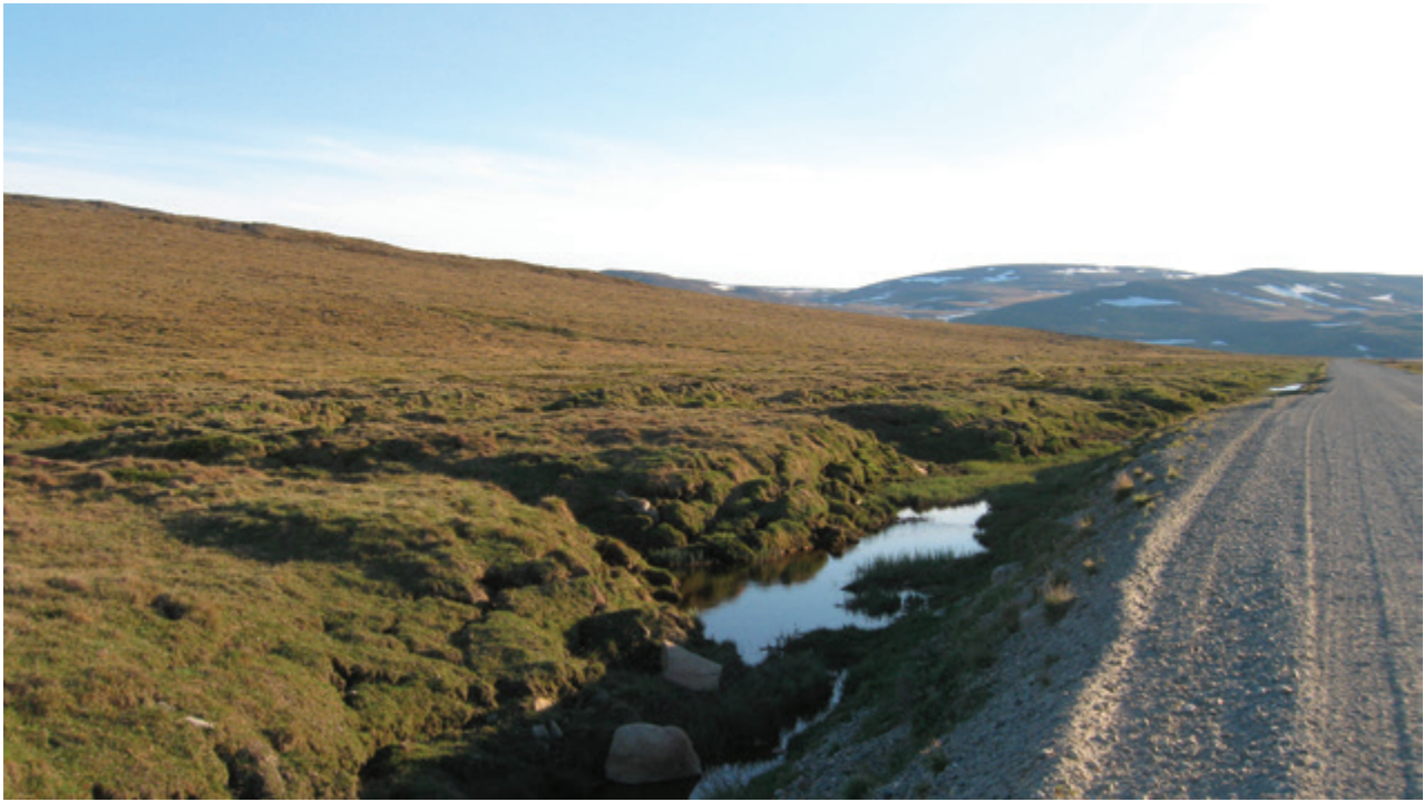
Figure 10.11 Water ponding in a depression created by thaw subsidence at the bottom of an embankment. This subsidence was facilitated by the thermal impact of a snow bank previously at the road's edge (photo by E. L'Hérault).
