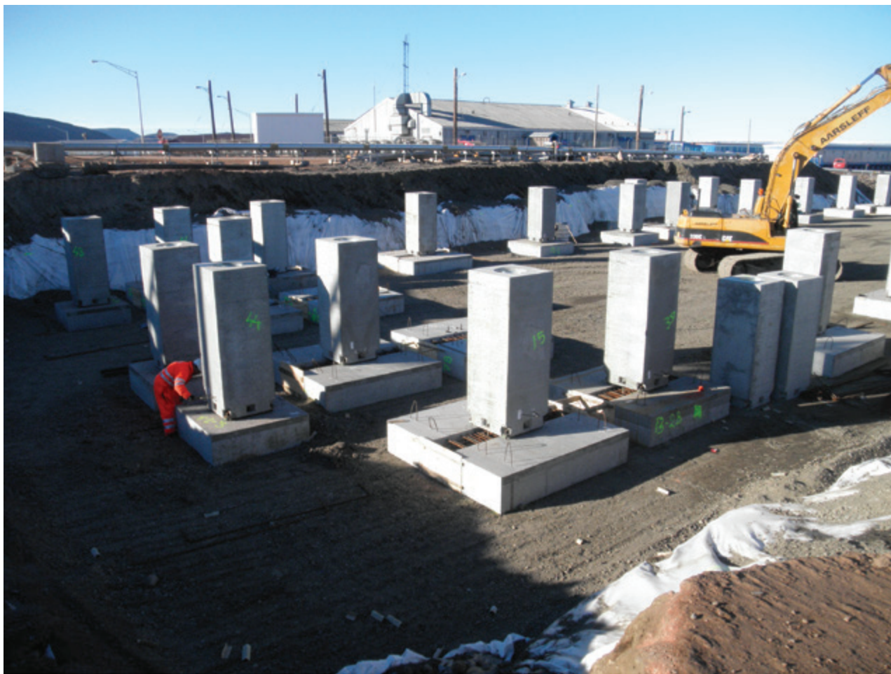
Figure 10.17 Excavation and placement of pier-and-footer style foundation for new dormitory, Thule Air Base (photo by Kevin Bjella).
