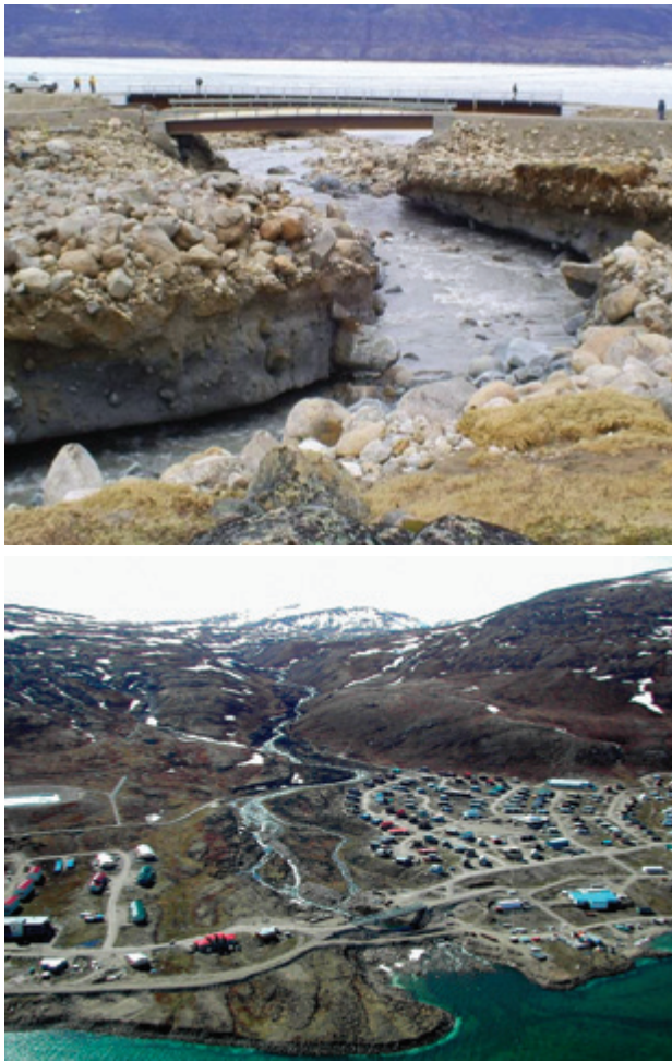
Figure 10.26 Extreme peak discharge of the Duval River in June 2008 resulted in downcutting of the riverbed, generating thermo-erosion and causing terrain collapse and the destruction of the Pangnirtung bridges (from Gosselin, 2013, and Carboneau, 2014).
