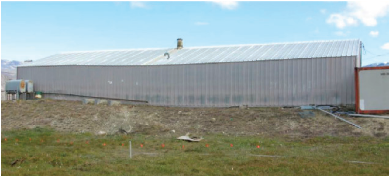
Figure 10.24 Municipal garage showing visible deformation (central depression) due to permafrost thaw settlement, Pangnirtung, Nunavut. Drillings next to this building revealed a very ice-rich surficial deposit (photo by E. L'Hérault).
