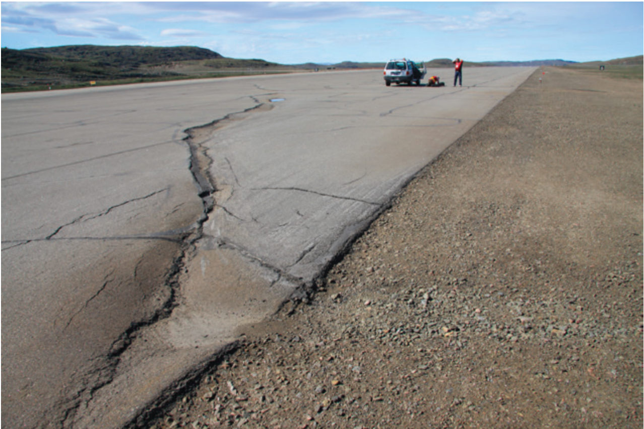
Figure 10.21 Linear depression caused by permafrost degradation at the Iqaluit airport (photo by E. L'Hérault).
