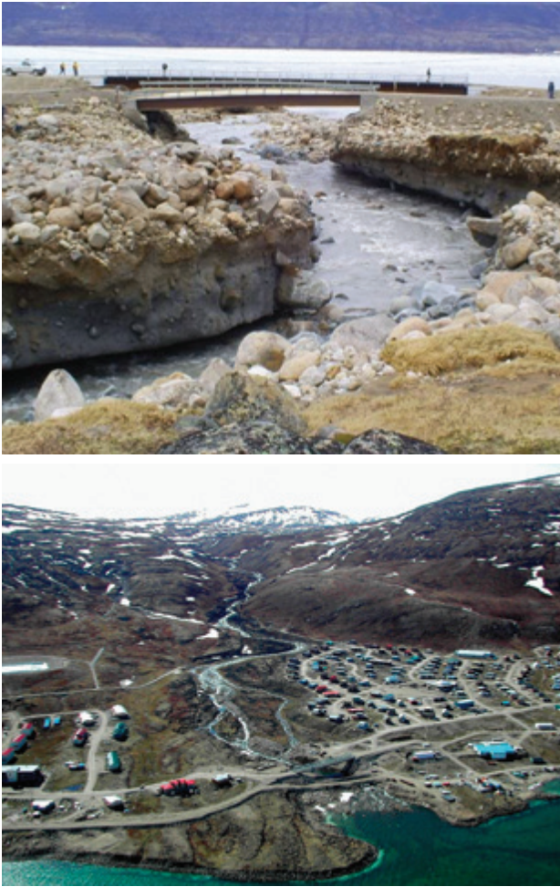
Figure 10.26 Extreme peak discharge of the Duval River in June 2008 resulted in downcutting of the riverbed, generating thermo-erosion and causing terrain collapse and the destruction of the Pangnirtung bridges (from Gosselin, 2013, and Carbonneau, 2014).
