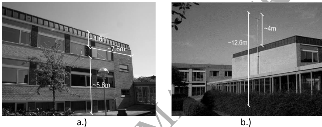
Figure 3. a.) Position of the office and the window opening in the full-scale experiments made at the office building. b.) Measurement of wind velocity and wind direction above roof level
