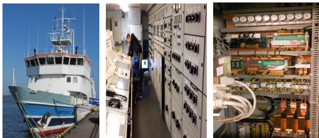
(a) Horyzont-II ship (b) engine room (c) control board
