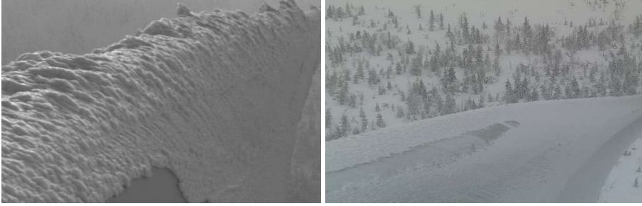
Figure 1.3: The pictures are taken from the hub and looking towards the tip of the blade. Left, the blade is heavily covered by ice and forced into standstill until the conditions change and the ice can melt. Right, the blade is covered by a layer of rime ice and is still in operation. The pictures from Stor-Rotliden wind farm were kindly provided by Vattenfall's Turbine Icing Program [7].
