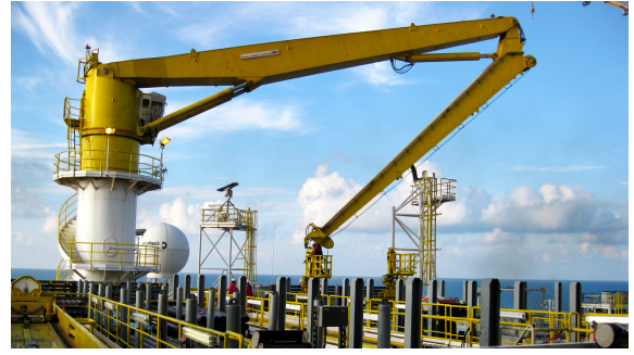
Figure 2: Knuckle Boom Crane example provided by National Oilwell Varco.©
