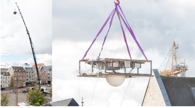
Fig. 2. Assembled setup lifted to 40 meters high by a crane (left) and zoomed (right)
