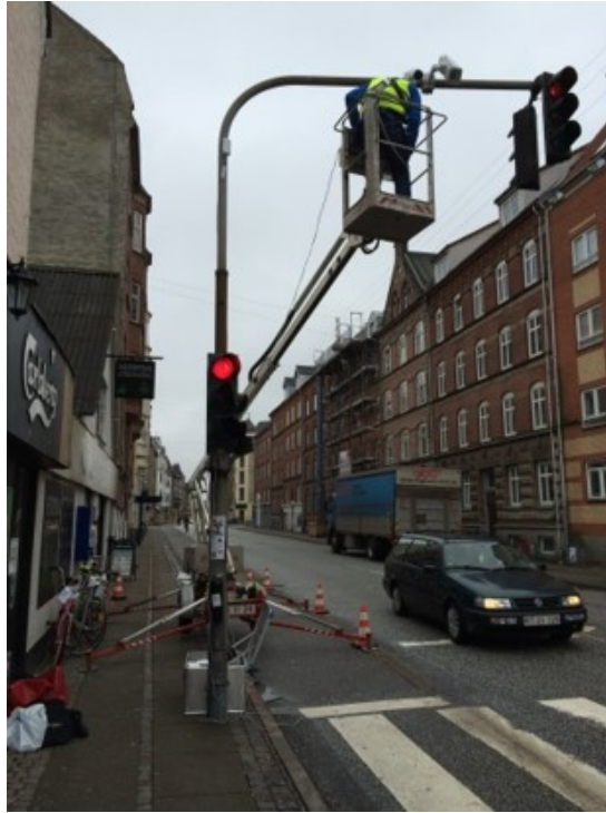
Fig. A.4: Cameras are installed in a traffic light pole. The cameras are connected NAS server inside the Eurobox located on the pavement next to the pole.
