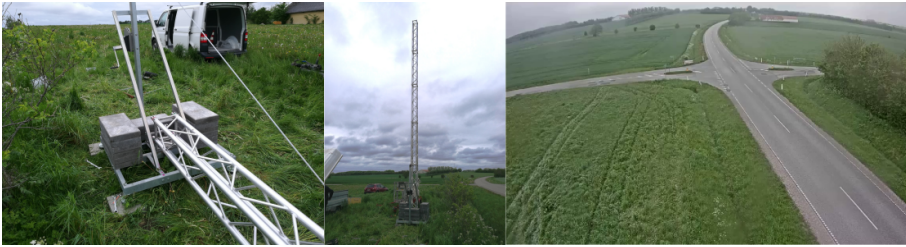
Fig. B.16: The TRG-pole is deployed at a traffic intersection with limited existing infrastructure.
