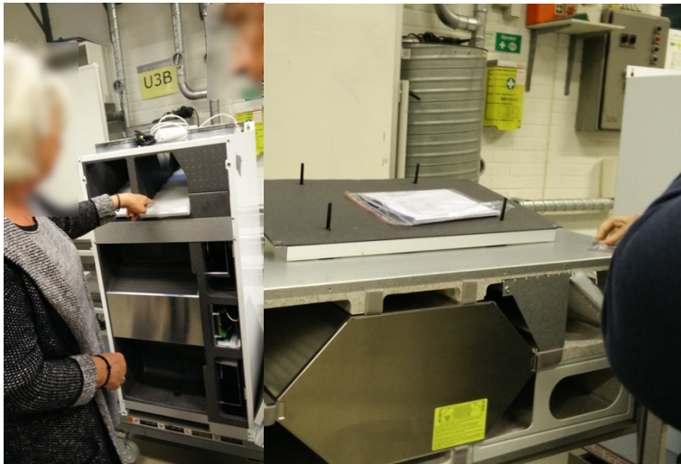
Figure 5.1: The estate board members look at decentralised ventilation units in the laboratory of an engineering consultancy company. The left picture shows how a board member points at the white filter in a unit. The right picture shows another type of unit.
