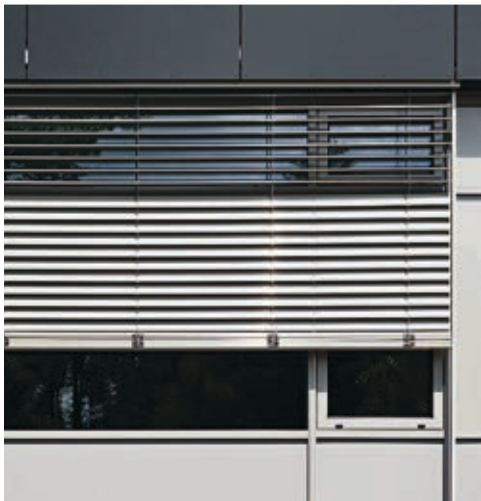
Fig. 25 Window with external solar shading that can be rear-ventilated. Source: C. Moosmann
