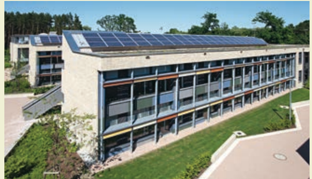
Fig. 27 Natural and mechanical ventilation is used in the Hohen Neuendorf demonstration project. Source: Ali Moshiri
