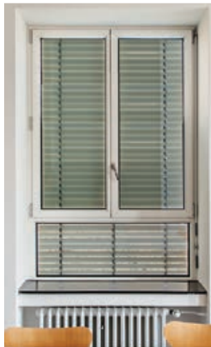
Fig. 26 Daylight situation in the room with external solar shading: l.) Completely closed solar shading; m.) Lower blind section closed, upper blind section with daylight control; r.) Slats in horizontal position. Source: S. Winterwerber, KIT
