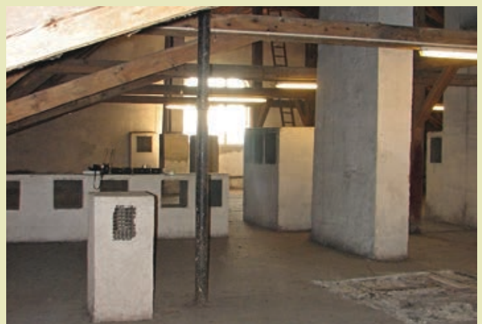
Fig. 16 Historic exhaust air stacks in the attic.
