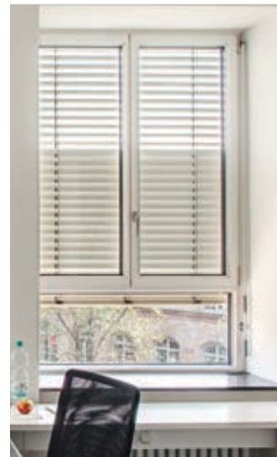
Fig. 26 Daylight situation in the room with external solar shading: l.) Completely closed solar shading; m.) Lower blind section closed, upper blind section with daylight control; r.) Slats in horizontal position. Source: S. Winterwerber, KIT
