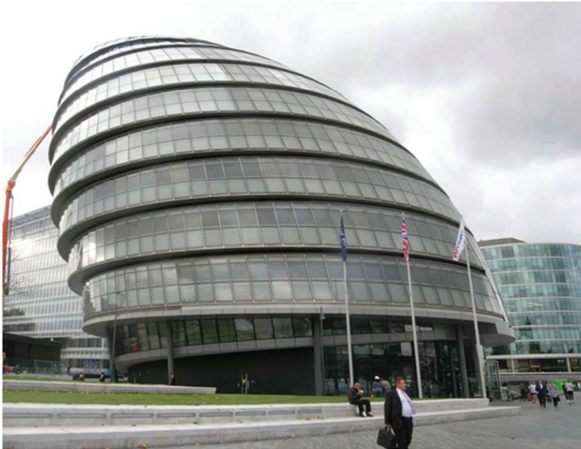
Photo 1. GLA Headquarter by Foster + Partners (Own photo)
