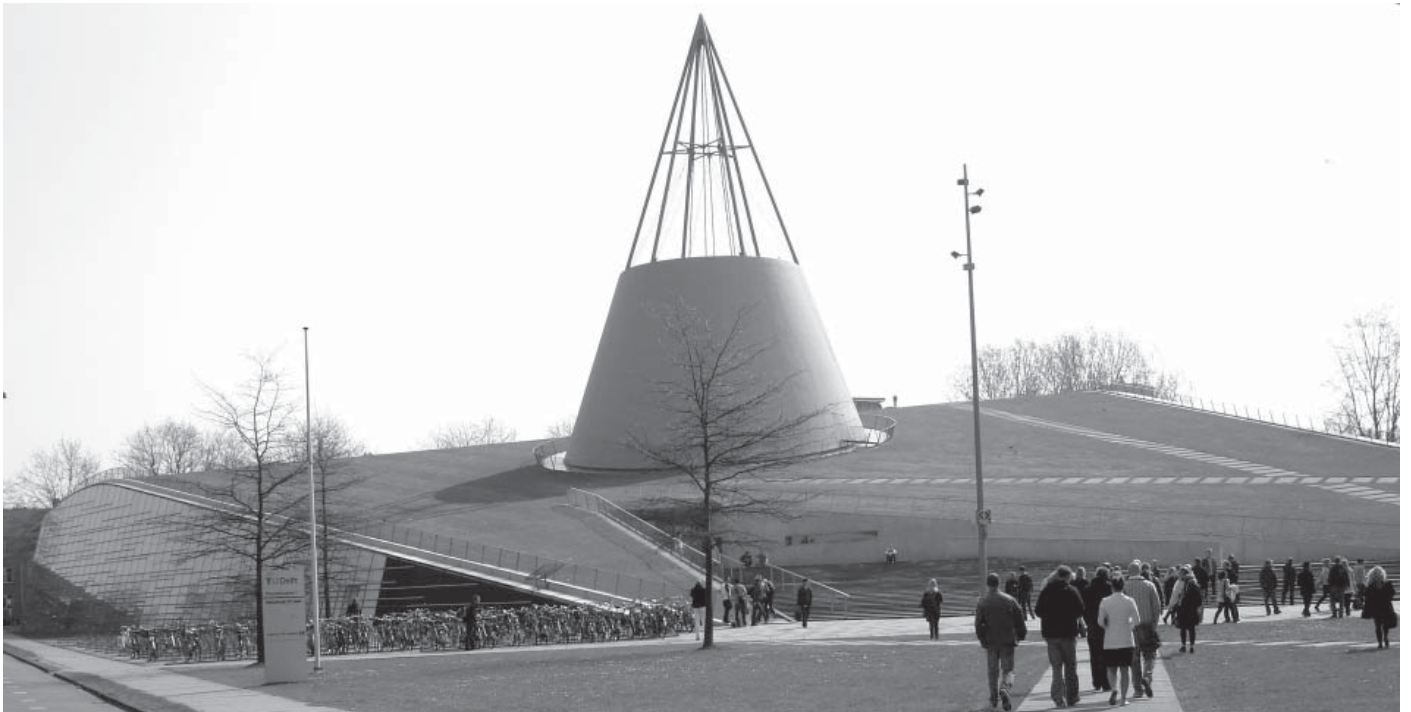
Fig. 14: Library in Delft by Mekano an example of an urban landscape approach (Photo: Lasse Andersson)
