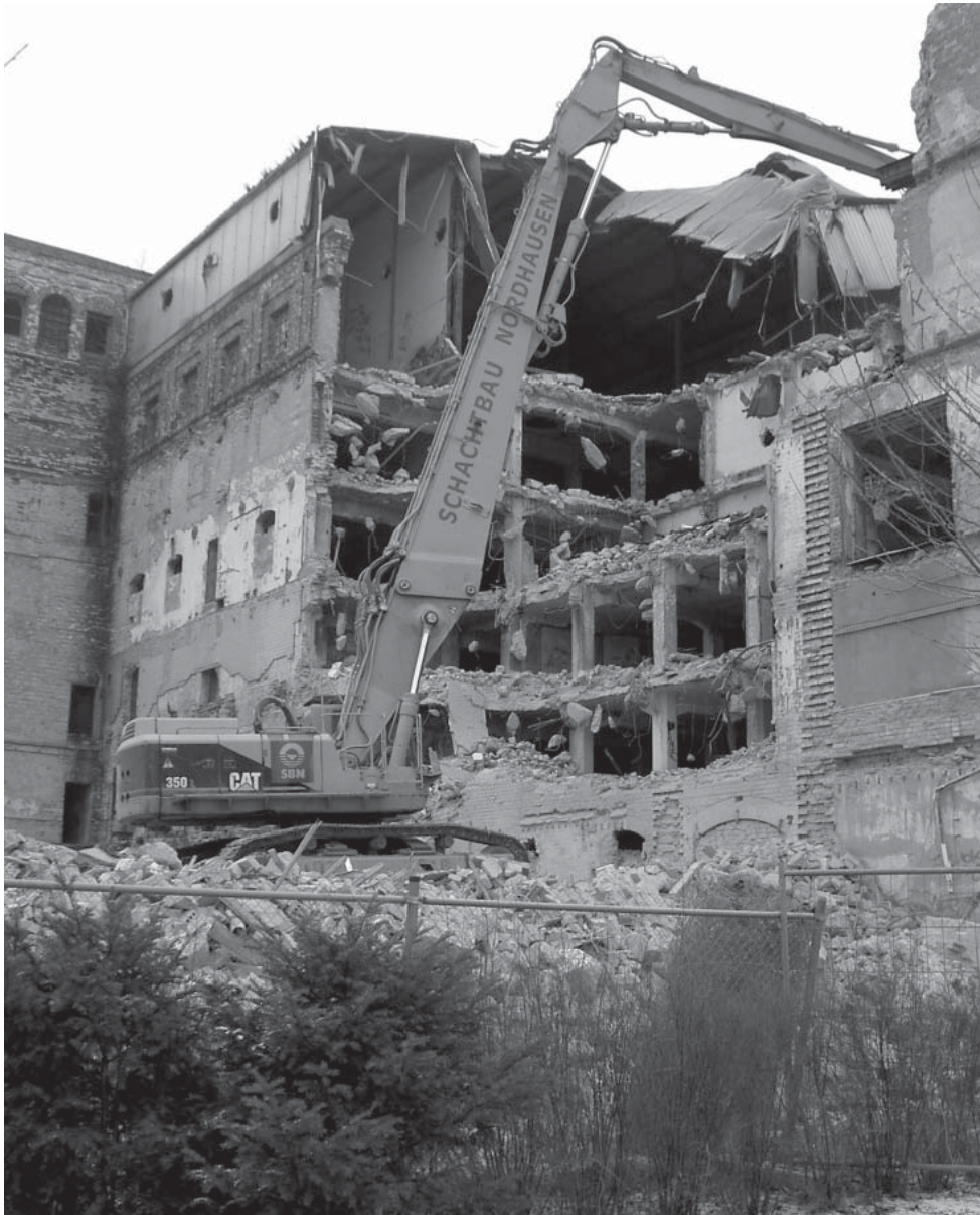
Fig. 20: Demolition of surplus buildings in Halle, Germany (photo: Lea Holst Laursen)
