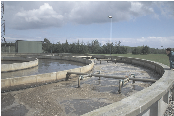
Figure 5.37 Part of the outer ring of the OCO tank during aeration.
