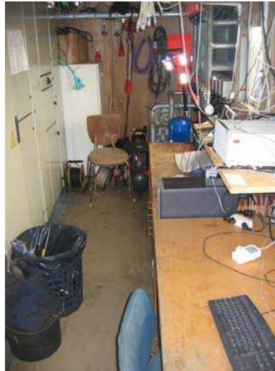
Fig. 6: Inside the control room of Wave Dragon, the PLC and Frequency inverters are in the cabinets to the left, in the far corner the piping, valves and blower for the automatic buoyancy can be seen, and to the right are the SCADA and data acquisition PCs in front of windows looking out onto the reservoir.
