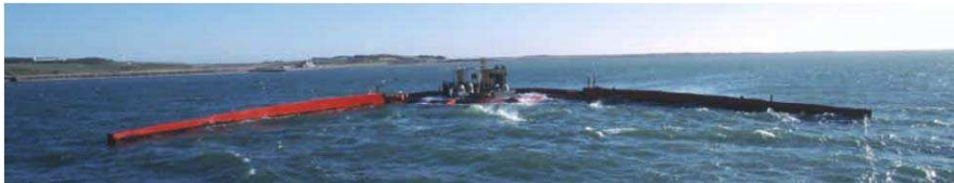
Fig. 1: The Wave Dragon prototype in Northern Denmark. The reservoir and ramp are situated in the middle, with the reflectors concentrating the waves towards the ramp.
