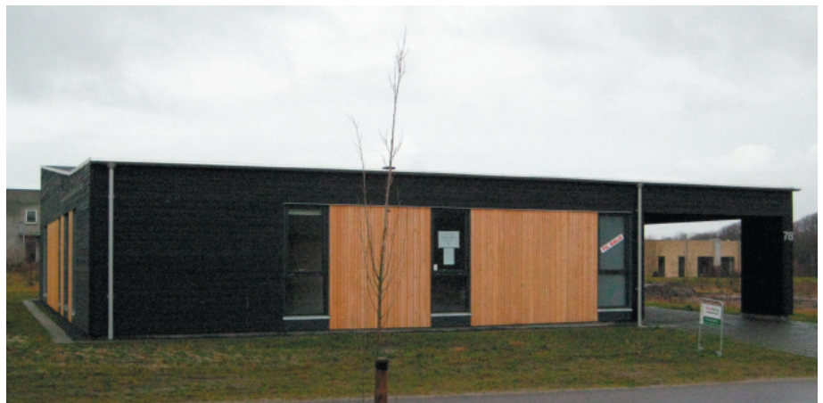
374. Contemporary prefab house constructed by 3D elements: The ONV house (M2 2008).
