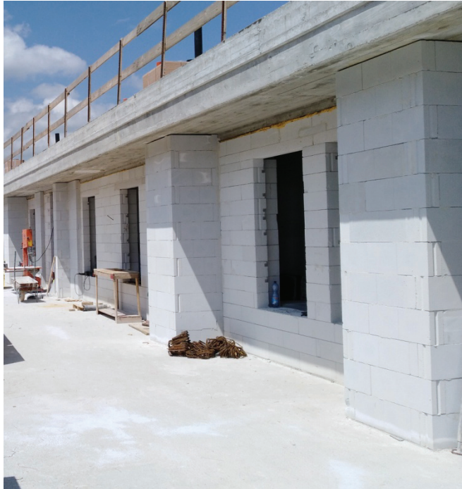
Figure 3.1: Facade built using the autoclaved aerated concrete blocks.
