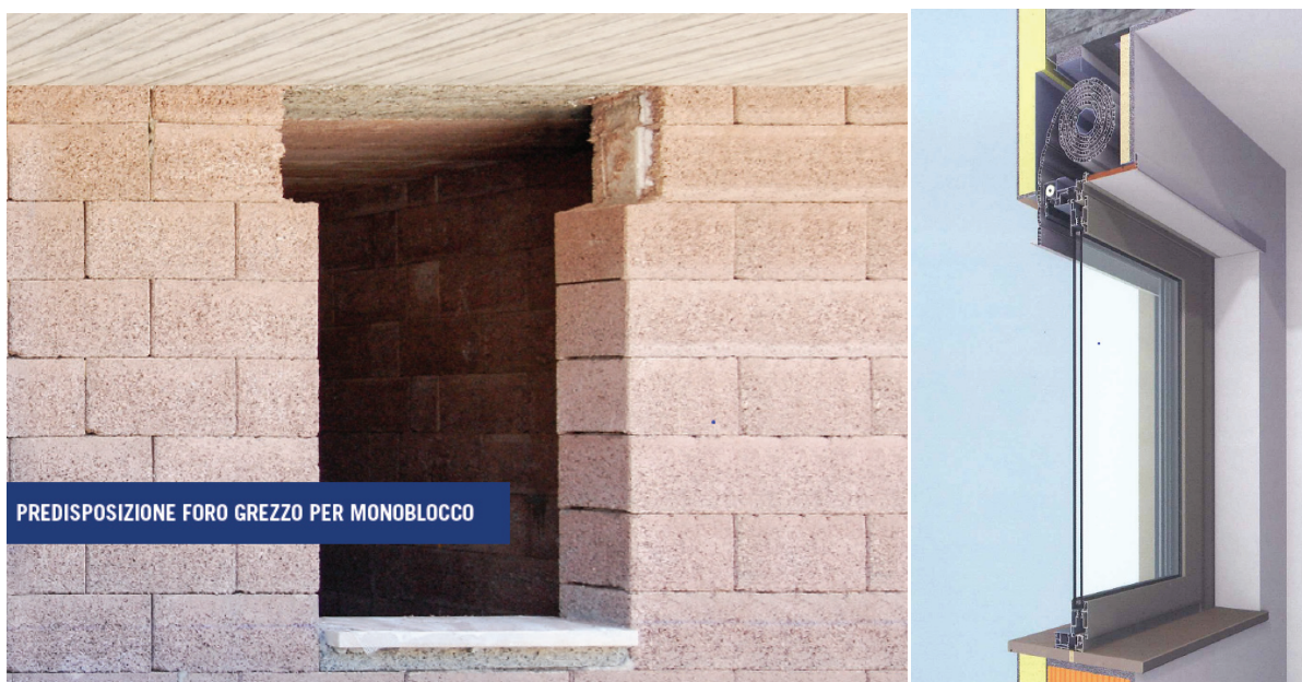
Figure 3.2: Hole in the whole for mono-block window, left, and a section of a mono-block window by Giulian srl, Italy
