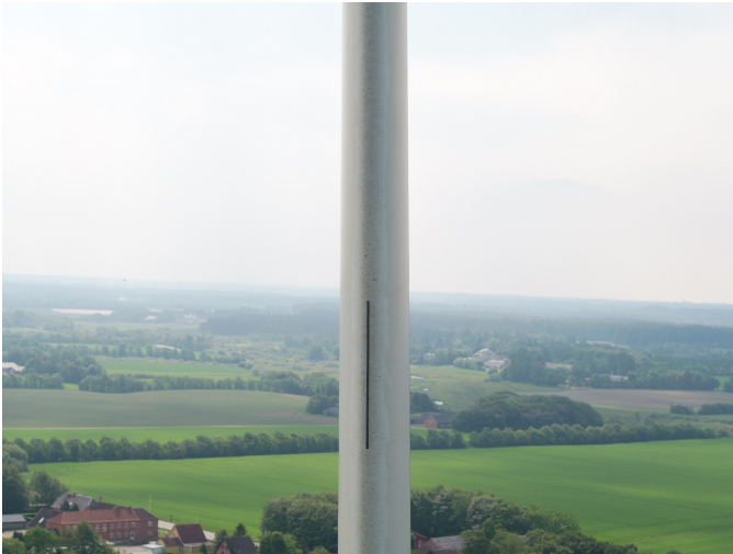
Fig. 10. Leading edge of the wind turbine, approximately 7 from the blade tip.
