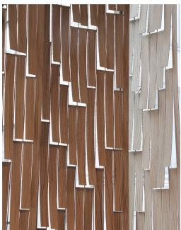
Figure 5 Full scale demonstrator with developed and tested thermal responsive composites in the Copenhagen School of Technology and Design Library. Left image shows the developed composite mounted in operable frames on the glass pane. Right side close-up of the composite bending and creating light permeability through the membrane.
