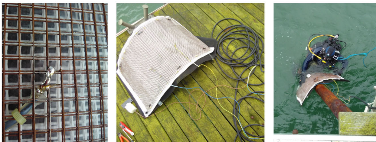
Figur 5. Electrodes installation at Nisum Bredning
