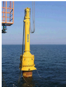
Up-close of installation of offshore piles ( www.4coffshore.com ).
