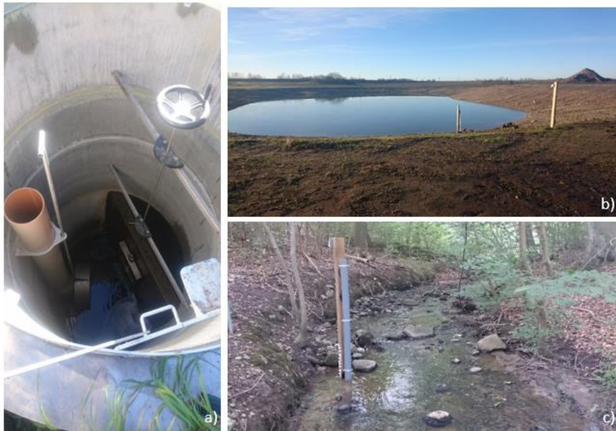
Figure 2.5: Measurement station in Aarhus (Beder Bæk). a) illustrates the water brake in the outlet from the detention pond, and b) illustrates the measurement station in the detention pond which discharges to Beder Bæk. c) illustrates the measurement station in the stream Beder Bæk.
