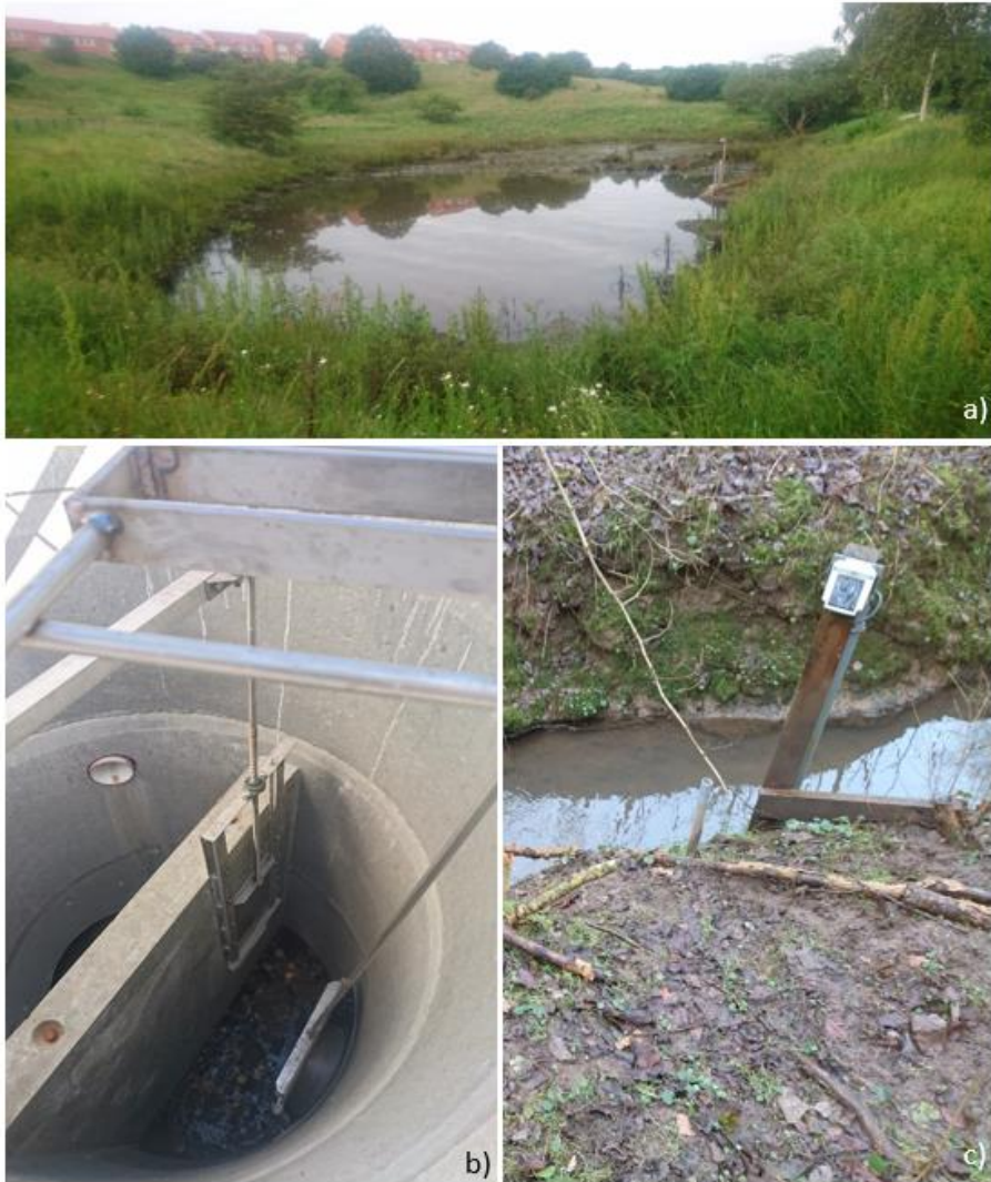
Figure 2.6: Measurement station in Vejle. a) illustrates the measurement station in the stream Polsterbæk. b) illustrates the sliding valve installed in the outlet from the detention pond which discharges to Polsterbæk, and c) illustrates the measurement station in the detention pond which discharges to Polsterbæk
