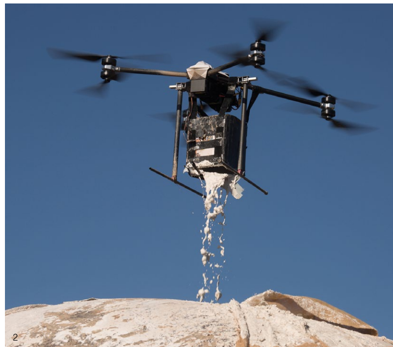
2. Drone depositing a coat over a large inflatable dome. Barcelona Drone Center, 2018. Photo: Frederic Carmona.
