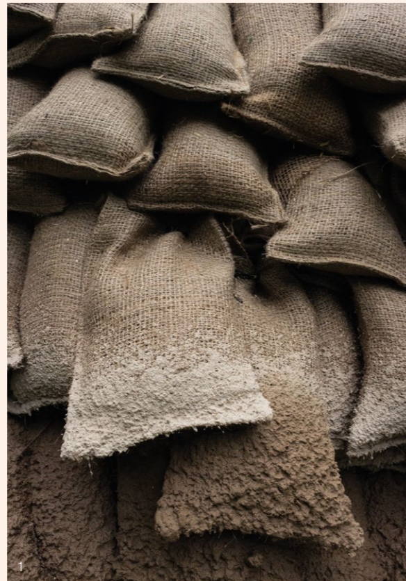
1. Jute bags filled with straw are arranged in a geodesic dome to be drone-sprayed with sustainable mortars at a later stage. Mud Shell project, London Design Festival 2018.
