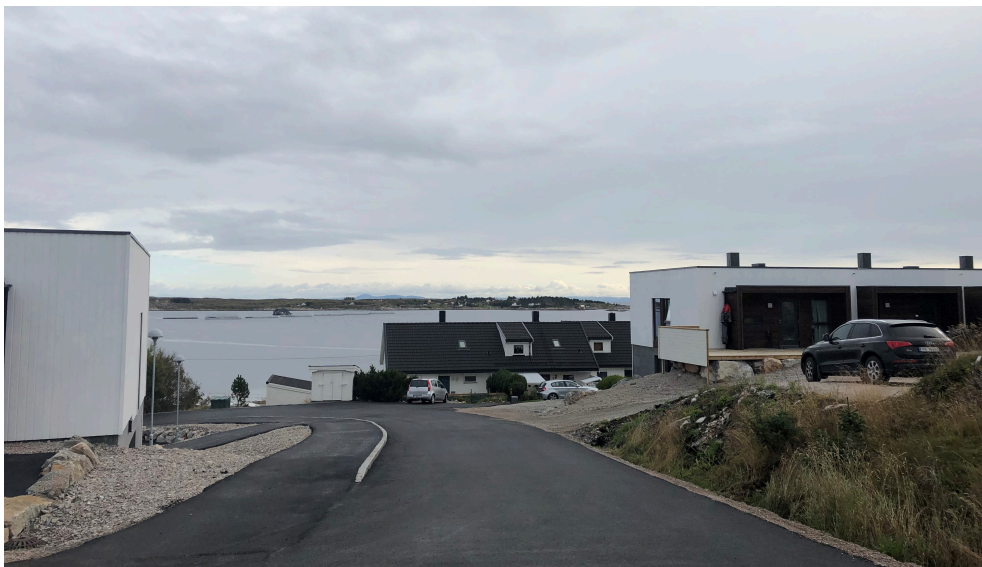
Newly-constructed terraced housing units in the city of Sistranda. Photo: Louise Ormstrup Vestergård.
