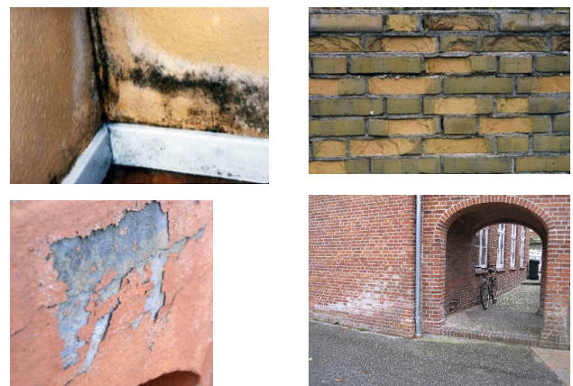
Fig. 3. Examples of visually apparent moisture induced damage of internal or external façades. From top left and clockwise: Mould growth at indoor surface, spalling due to frost, salt efflorescence, scaling of paint.
