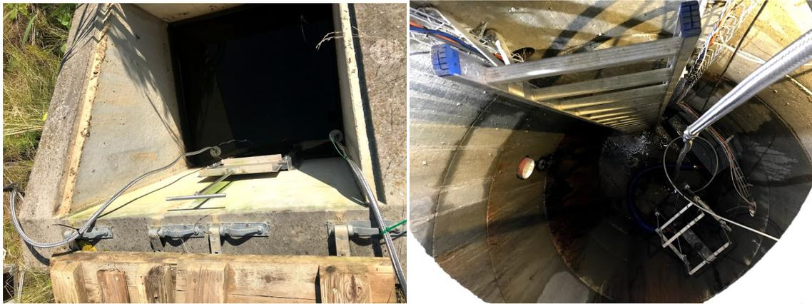
(a) Soil filter system inlet water sampling point (Stormwater pond outlet) (b) Soil filter system outlet water sampling well
