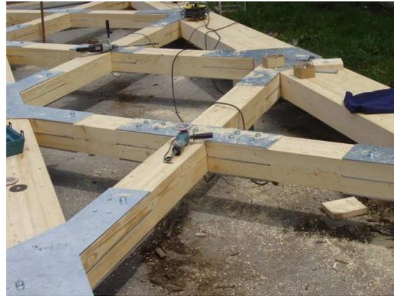
Figure 3: Details of tensile and compressive elements
