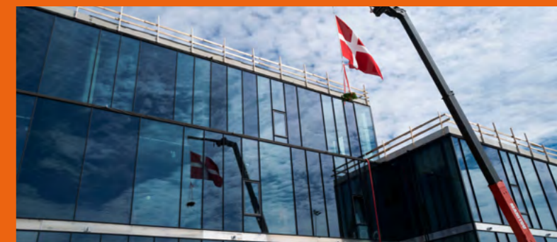
Topping-out ceremony, AAU Science and Innovation Hub, 2021 (Photo: Lars Horn, Baghuset)
