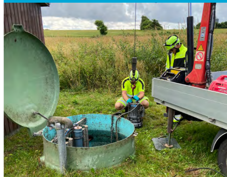
In the SWIFT project, pumps for wastewater management require continuous scrutiny and maintenance. Remote sensing technology collects and transmits real-time data from the utility networks, aiming to lower the risk of wastewater pump clogging (Photo: Jonas Falzarano Jessen)
