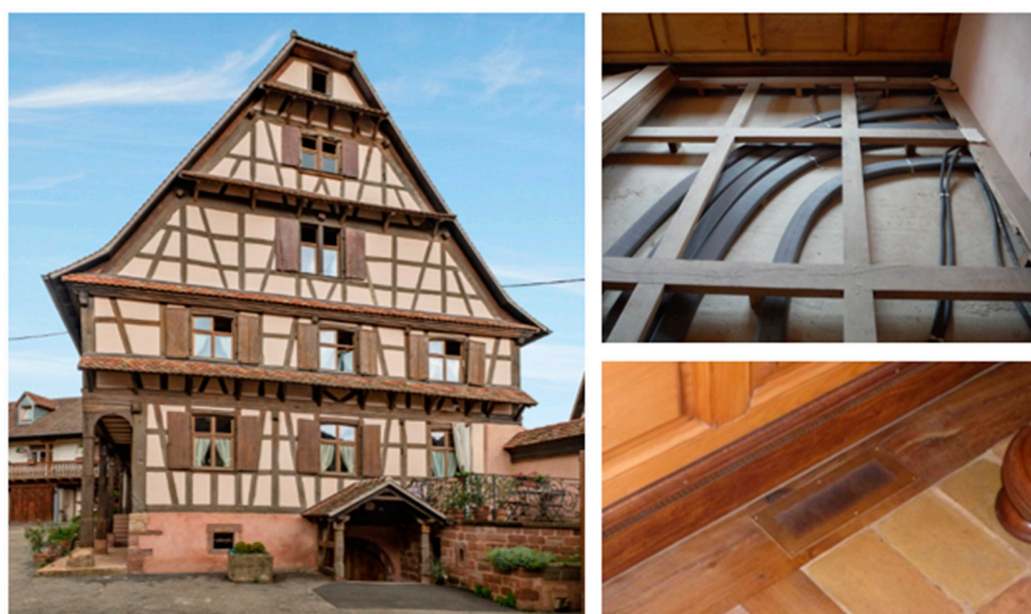
Figure 2. One of the documented examples. A timber-framed house from 1783 in Schnersheim, Alsace, France: Architecture, a “hidden” air supply, ventilation ducts of the HRV in the floor. Source: Denis Elbel.
