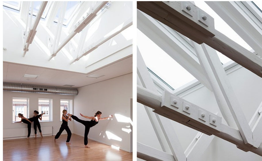
Figure 16. The roof lights provide a significant amount of daylight to the first floor in the building.
