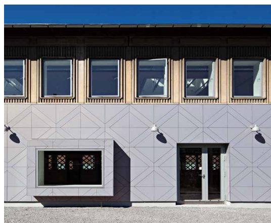
Figure 6. Façade facing the garden after renovation.
