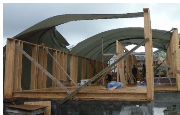
Figure 4. Windy conditions at building site during summer.
