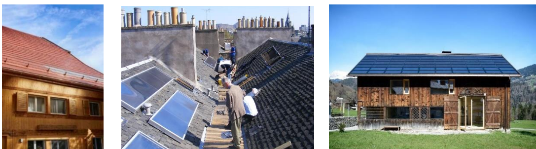
figure 5: left: colour modules terracotta of PV © Solaragentur Prix Solaire Suisse 2018, Maison rurale Galley, 1730 Ecuwillens/FR; middle: solar thermal units on ten protected blocks of flats in the City of Edinburgh. © HES; right: side view of the House Breuer (Austria) with non-reflecting PV modules with a dark background ©FG Marcello Girardelli
