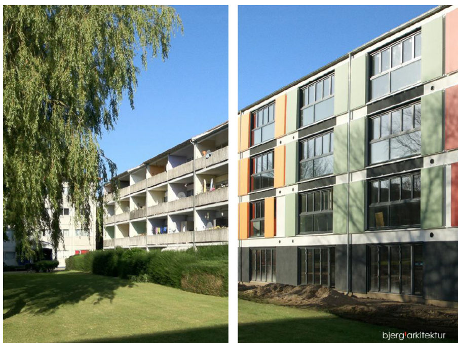
Fig. 3. Balconies of Gadehavegård before (left) and after (right) renovation (Photos: Bjerg Arkitektur).
