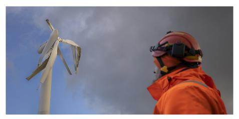
Fig. 1.7: The Nordtank wind turbine strucked by lightening. Photo by B. Á. Rubeksen.
