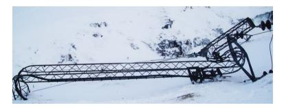
Fig. 1.4: A transmission tower after a heavy winter storm.
