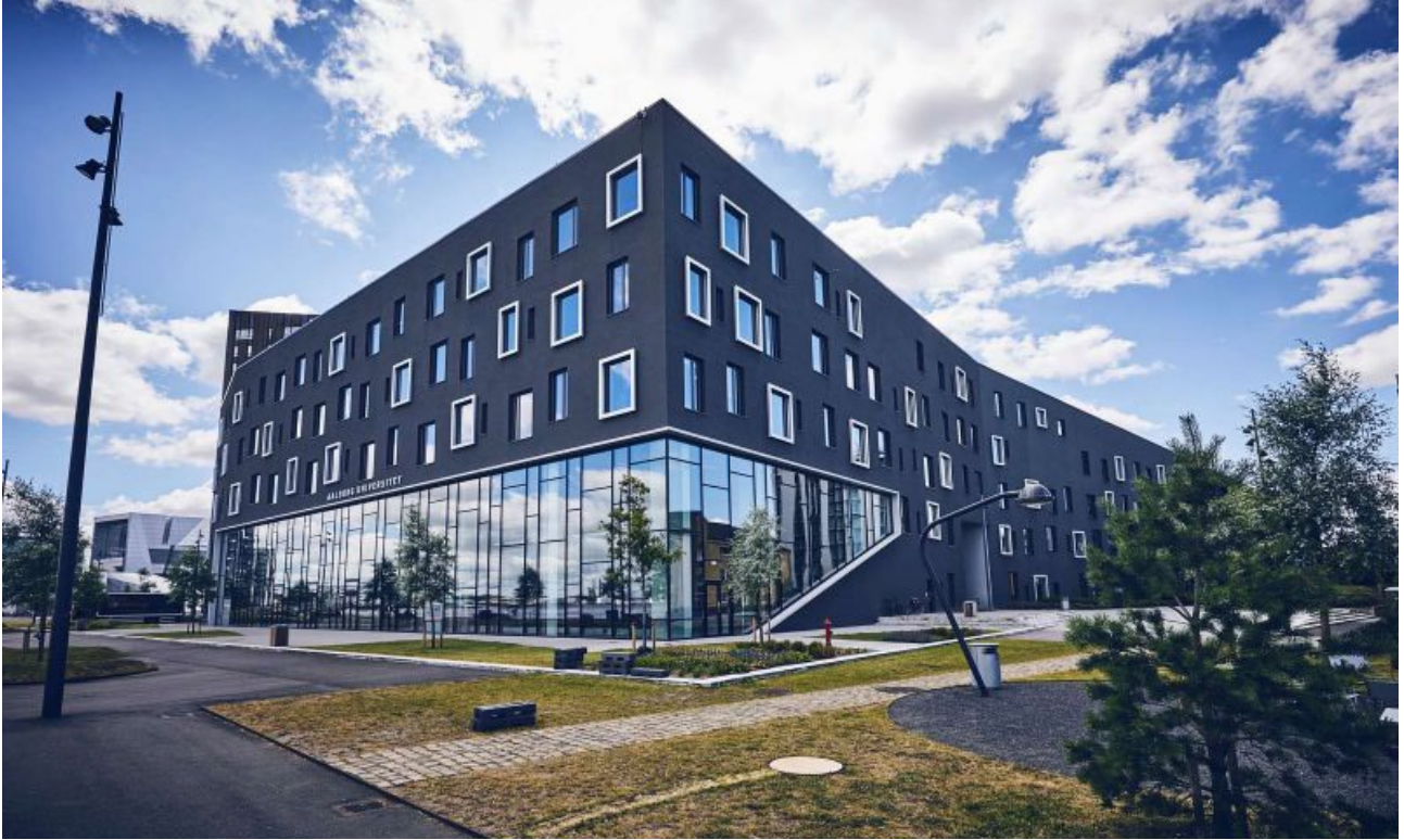
Figure 3: View of the building study case: CREATE - Rendsburggade 14, 9000 Aalborg, Denmark.
