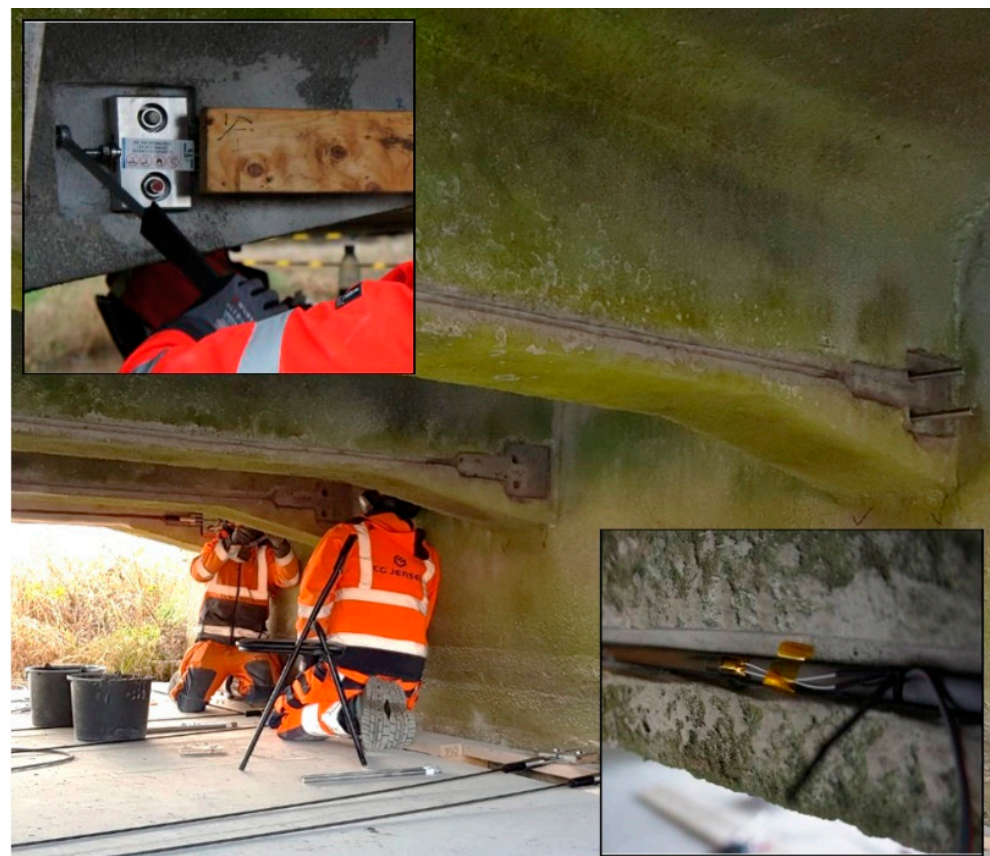
Figure 16. Site installation of the throughgoing threaded bar and pre-stressing of the system. Photograph by S&P.
